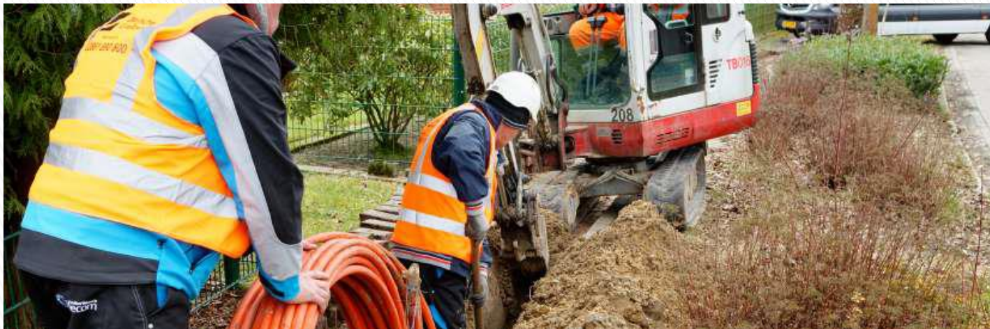
Figure – Protected microduct laid in open trenches
