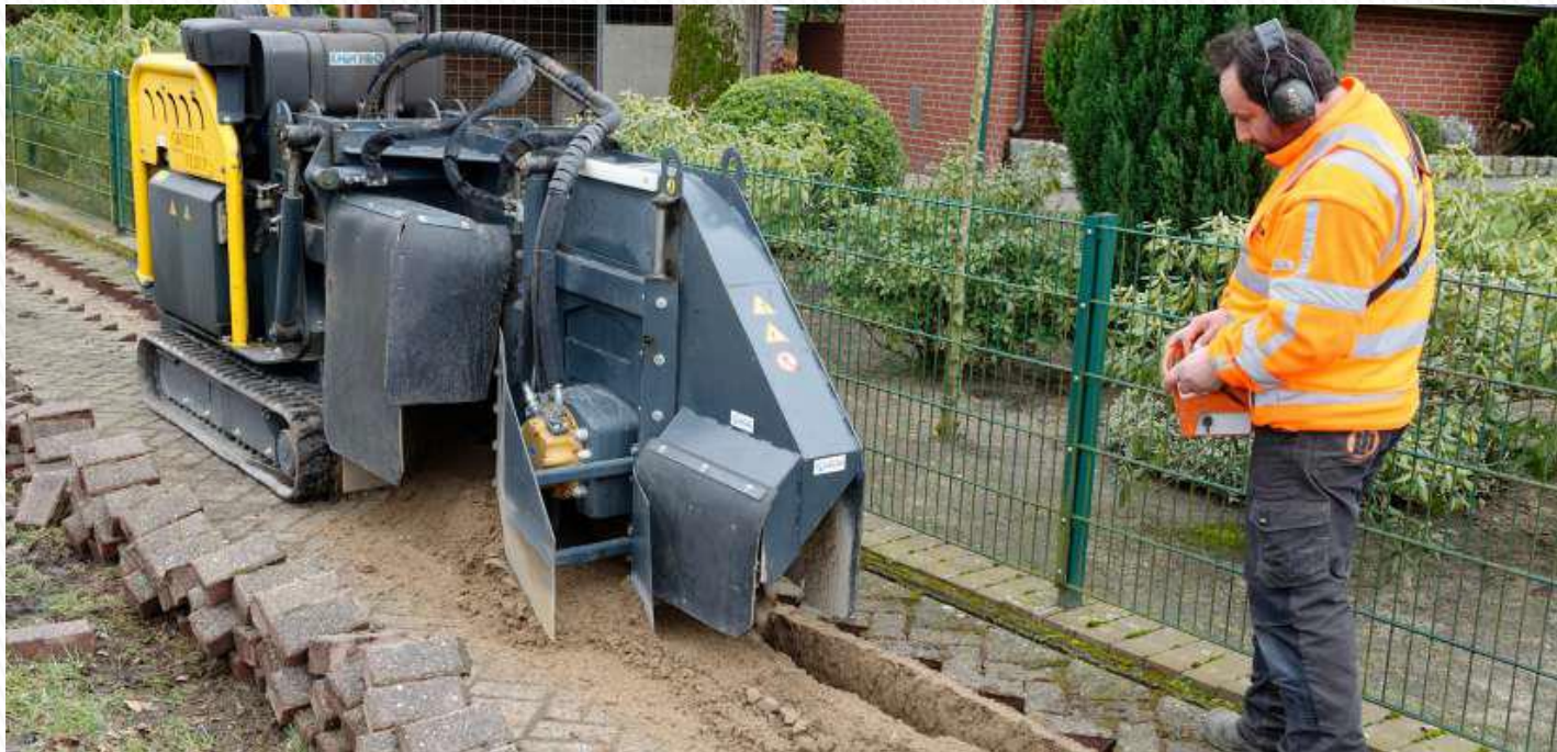
Figure - Micro trenching deployment technique
